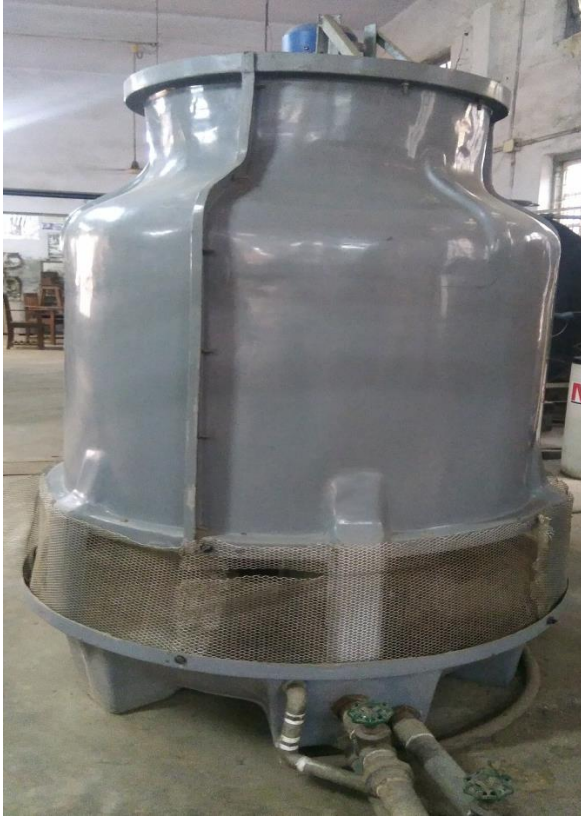
Modular Cooling Tower
